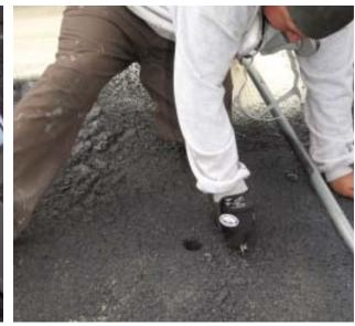
Figure 4. Although some sheet metal can be reused, scuppers (above) and drains should be replaced so the foam has a clean surface to bond to. Here, a roofer cuts out the membrane around an existing drain (above right); it's replaced with a new dropout fitting (right) that feeds to a downspout below. The new fitting will be nailed to the deck and primed before the foam is applied.
