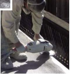
Figure 7. The applicator pulls up on the masking paper while spraying foam up and onto the edge metal (above left). After spraying such detail areas as edges, curbs, and roof jacks, he sprays the main body of the roof (above). A worker uses a grinder to bring the foam flush to the edge metal (left) and to make it slope properly into scuppers and drains.
