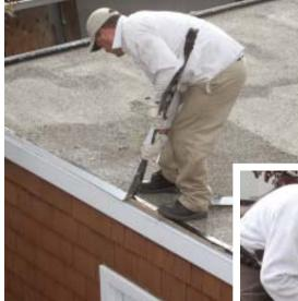
Figure 3. Before SPF is applied, the existing gravel stop is removed (above) and replaced with a new stop designed for foam. The crew uses polyurethane sealant and at least two nails at every lap (right) to prevent the joints from flexing and cracking. Next, the stop is nailed 9 inches o.c. to the edge of the roof.
