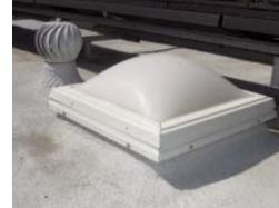
Figure 6. The crew takes skylights off the curbs before applying foam. This curb will be too close to the surface after the foam is applied, so the roofers extend it with a wood frame (above left). Then they mask the opening and waterproof it with a layer of foam (above). Once the rest of the roof has been foamed and coated, they remove the masking, apply weather-stripping to the curb top, and reinstall the skylight (left).
