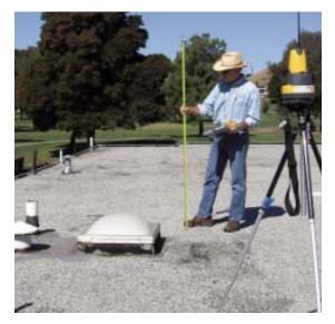
Figure 1. The author uses a laser level to measure the elevation at various points on the roof (above) and then records the information (right). The map tells the applicator where the low spots are so he can build up those areas with a thicker layer of foam and thereby prevent ponding.
