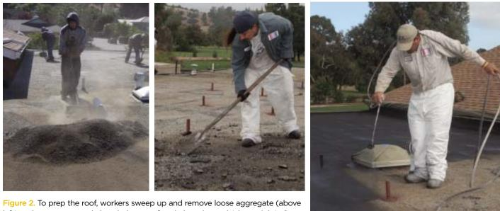
Figure 2. To prep the roof, workers sweep up and remove loose aggregate (above left) and scrape up poorly bonded areas of asphalt and gravel (above right). Once the roof is clean, they spray on a primer to make the foam stick better (right). The vertical posts — which were just installed — will be used to support solar panels.
