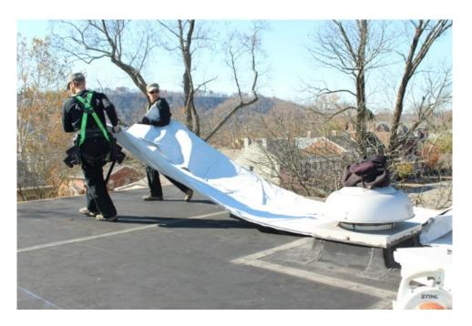
Covering a black rubber roof with a with white PVC membrane can reduce roof top temps by 50 to 80 degrees meaning an over all summer time cooling saving of up the 15%
