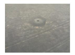
that moisture has entered under the rubber membrane and deteriorated the adhesive that glues the rubber to the insulation board. The rubber wrinkles as it is no longer glued down in that spot.
