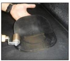
3) Apply the Uncured PS tape to the primed area. Once fitted cut a small section from the centre of the tape out to expose the outlet opening and press the remaining tape down into the outlet. Roll the entire flashing with hand roller.
