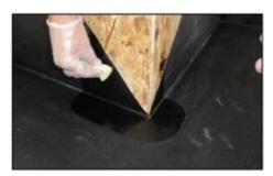
2) Apply Primer to the marked area to be flashed and allow to dry. The area must be clean and dry before application of primer, apply primer to membrane and to upstand substrate. Primer must be allowed to dry before application of tapes.
