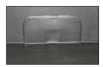
2) Install the EPDM membrane over the outlet with Bonding Adhesive. Do not apply adhesive to 50mm section around outlet opening.
