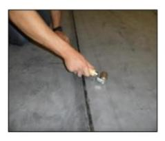
4) After the entire seam is put together, roll the entire length of the seam with a steel or silicone hand roller. Roll the seam at right angles to the seam direction, not along it.
