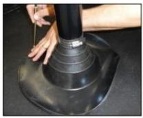
Once in position clamp the seal to the pipe with the supplied metal clamp and mark around the base of the seal to give a line to prime up to. Pull pipe seal upwards on pipe to expose the membrane.
