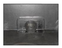
7) Once the second section of tape is installed, complete by inserting the leaf grate into the outlet.
