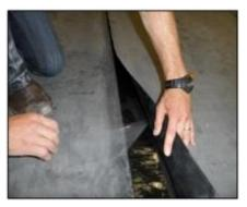
3) Lay the top membrane onto the Seam Tape poly backing. (If the Seam Tape does not visibly extend beyond the edge of the top membrane, the membrane edge should be cut back to expose 5mm (1/4") of Seam Tape.
