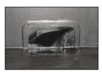
4) Install Uncured PS tape to the outlet. This should be large enough to join onto the membrane by a minimum of 50mm.
