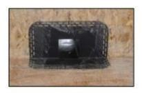
1) Install outlet into parapet wall before installing EPDM membrane.
