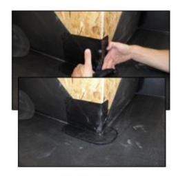
7) Work the tape onto the deck around the corner and smooth out.
