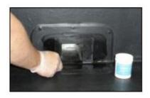
3) Cut the EPDM membrane away from outlet opening by 50mm. Apply Primer to the membrane, outlet face and into the outlet pipe.
