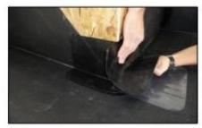
9) Repeat the process from the other direction, applying the primer and overlapping on top of the first corner detail.
