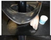
3) Apply EPDM Primer to the EPDM deck membrane in the area where the base flange will be bonded. Allow to dry.
