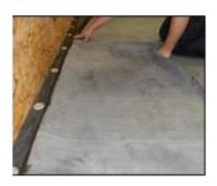
3) Lay the primed membrane into the PS tape with no wrinkles or air gaps and smooth in by hand.
