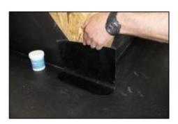
1) Cut the EPDM membrane at 45° angle to allow the membrane to run around the corner and create both upstands. Bond in place with Bonding Adhesive. Cut a section of 225mm Uncured PS tape to the required size and mark around it (min. 75mm onto deck, 75mm to turn round corner and 50mm past angled cut in membrane).
