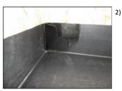
The fold should be cut back to leave a 75mm wide flap. Apply EPDM Primer to the front & back of the flap and to the membrane on the wall. The Primer must be allowed to dry before application of PS tape.
