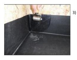
Cut an appropriate size piece of 225mm uncured flashing (min. 50mm wider than the flap of membrane), press the flap back to the upstand and install the uncured flashing tape. Roll the taped area with hand roller once installed.
