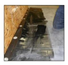
2) Apply the Bonding adhesive to the side of the RUSS strip or exposed decking. Also apply the Bonding adhesive to the relevant upstand termination or step down and to the back side of the material.
