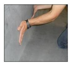
4) Apply positive pressure to the membrane to achieve a strong bond between membrane and required surface.
