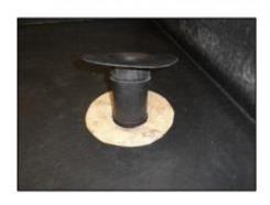
1) Cut the outlet flange back to leave a min. 50mm head and cut the membrane back to meet the perimeter of the outlet head.
