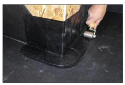
10) Once the second section is installed roll the entire flashing with hand roller.
