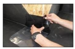
4) Fold the 75mm return of tape round the corner and press into position and work down so the bottom of the tape is a finger width from the deck.
