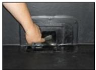
5) Cut a small square out of the middle of the tape and mould the tape into the outlet pipe by 25mm.
