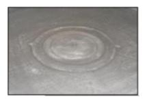
Fit the outlet into the roof before installing the membrane; ensure the outlet has the yellow protective cap installed. Install the EPDM membrane to the roof and over the outlet.
