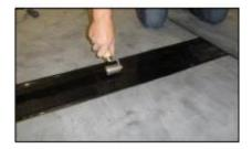
4) Once the entire length of tape is applied to the seam, roll across the 150mm tape with hand roller. Where 150mm
