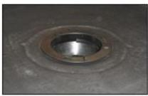
6) Screw in the clamping ring till it's completely tightened.
