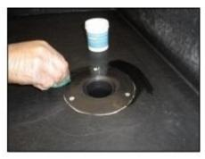
Secure the outlet into the decking and apply Primer to the head of the outlet and to the EPDM membrane.
