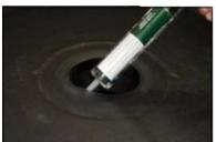
4) Insert a bead of ClassicBond Water Cut Off mastic between the underside of the membrane and the top flange on the outlet.
