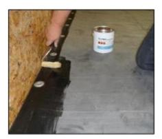
Once the flat area has been adhered using deck adhesive, keep the 100mm area around the perimeter free from glue. Fold back the sheet material to expose the clean deck area, upstand and the rear side of the membrane sheet.
