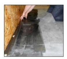
3) Mate the two surfaces together leaving no voids between the membrane and the receiving surface.
