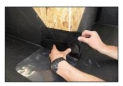
Once the Primer has dried, start installing the tape from the top point. Work the tape down the main face first; make sure no air is getting trapped.
