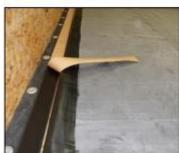
2) Once the primer is dry remove the protective strip from the PS tape on the RUSS strip.
