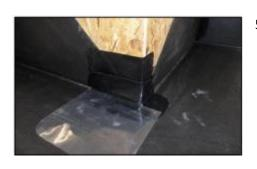
5) Work the tape down into the angle change, removing any trapped air. Using the clear poly lining to prevent contact to the deck will help when doing this.
