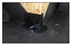
6) Fold the tape onto the deck on the longest side until 75mm from the corner and then fold the short side onto the deck.
