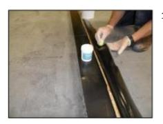
1) Fold the top sheet back to expose the seam area. Using a scrubbing pad apply the Primer to the seam area with back and forth strokes & moderate pressure until the seam surface attains a smooth black appearance. Apply the Primer past the seam edge to the chalk line. Primer must be dry before application of PS tapes.
